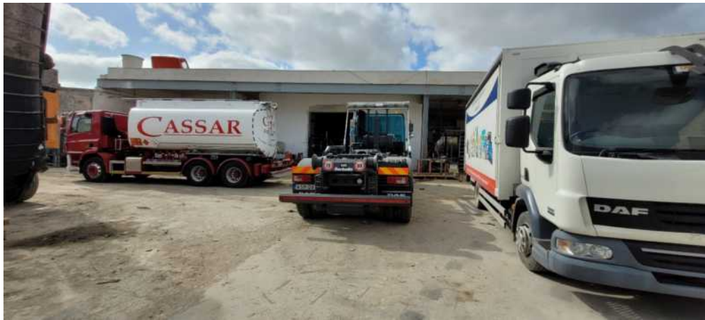
Figure 45 – Street Level; First portion, with frame structure in the background and third portion in the foreground with parked vehicles
