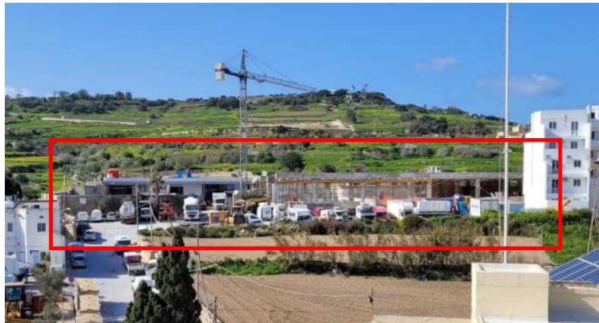
Figure 41 – Elevation of the Property in Subject as seen from Bonnici House
