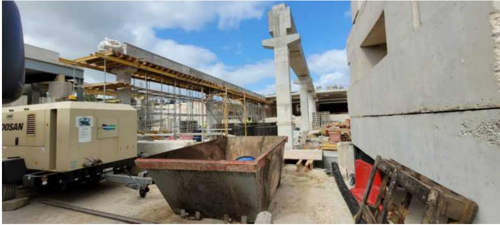
Figure 48 – Street Level – Second portion under construction
