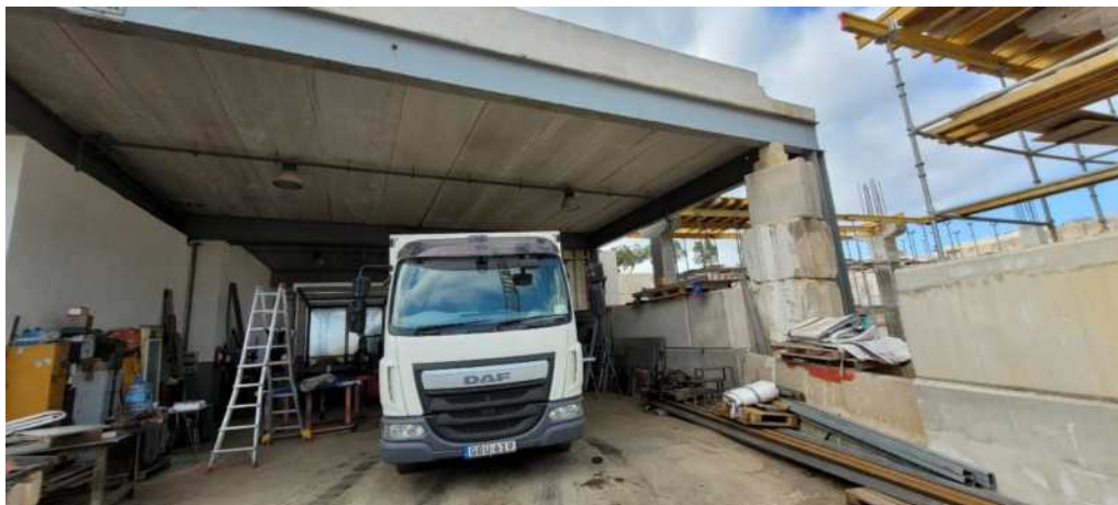
Figure 47 -- Street Level; Existing portal frame structure
