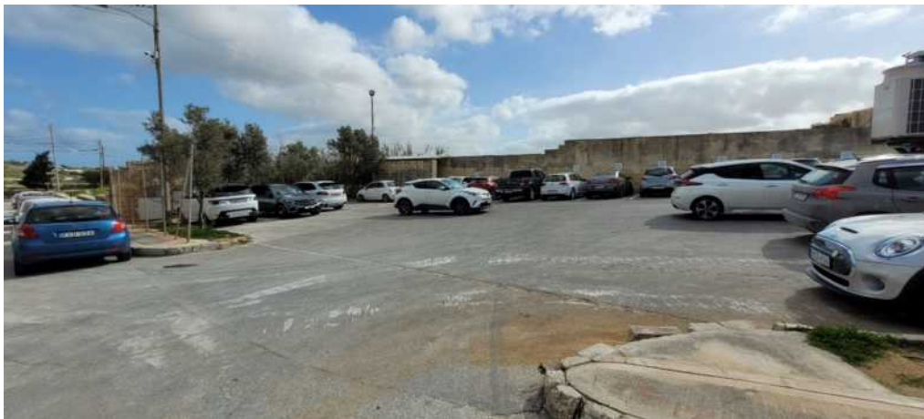
Figure 29 –Property in Subject off Triq is-Sardin
