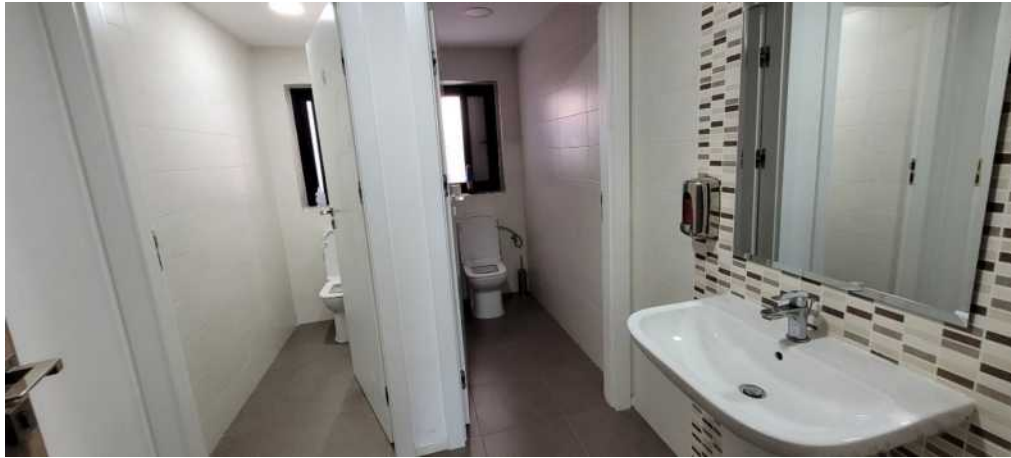
Figure 14 – Int; Typical Communal Bathrooms
