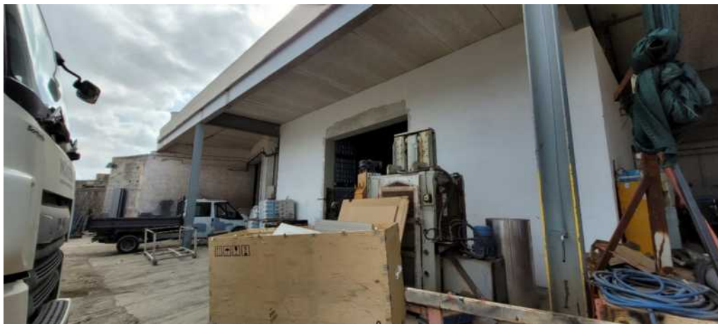
Figure 46 – Street Level; Existing portal frame structure
