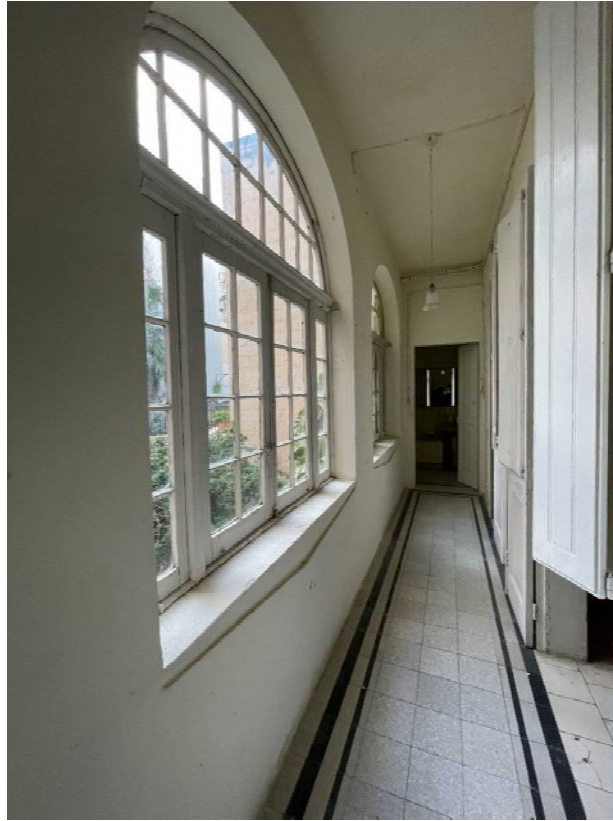
Figure 69 – Int; First Floor corridor overlooking backyard
