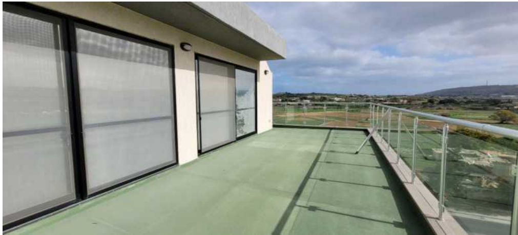
Figure 18 – 4 th Floor Level; Outdoor terrace at Penthouse Level
