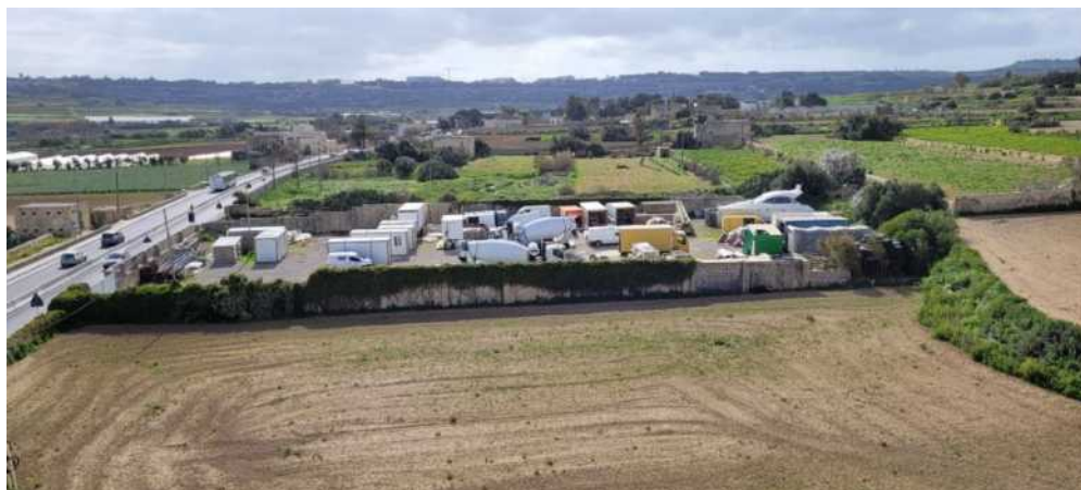
Figure 52 – Elevation of the Storage area of the Property as seen from Bonnici House
