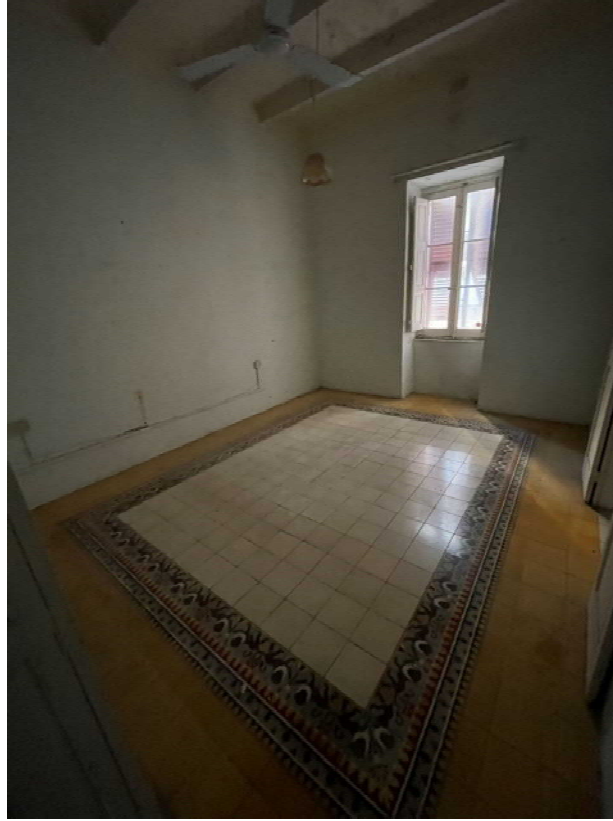
Figure 68 – Int; First Floor Bedroom
