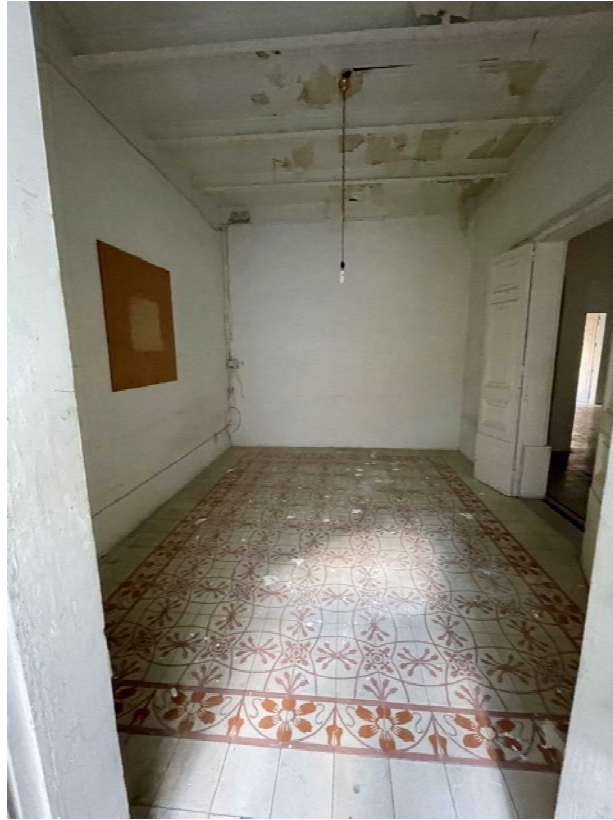
Figure 70 – Int; First Floor internal room
