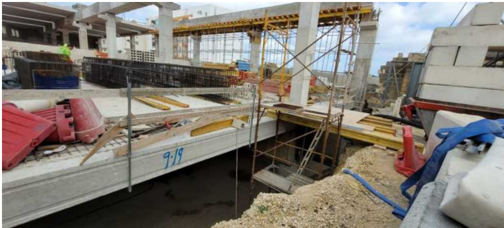
Figure 49 – Street Level – Second portion under construction with underlying basement level
