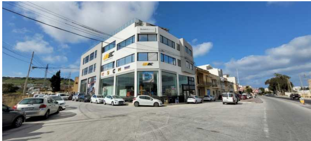
Figure 4 – Elevation of the Property in Subject at the corner of Triq is-Sardin with Triq Burmarrad
