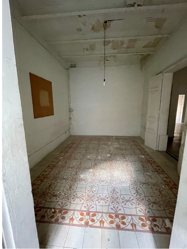
Figure 70 – Int; First Floor internal room
