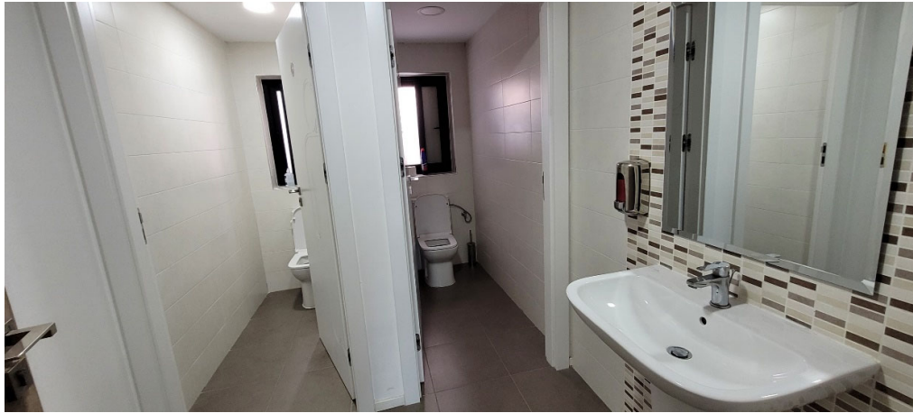
Figure 14 – Int; Typical Communal Bathrooms
