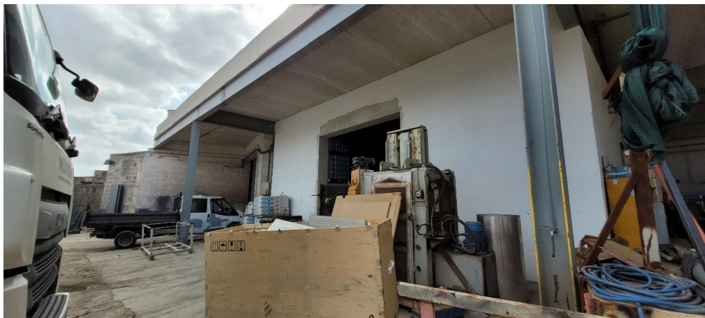
Figure 46 – Street Level; Existing portal frame structure
