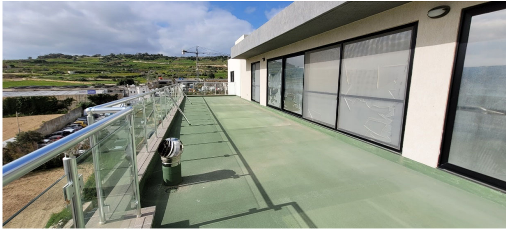
Figure 17 – 4 th Floor Level; Outdoor terrace at Penthouse Level
