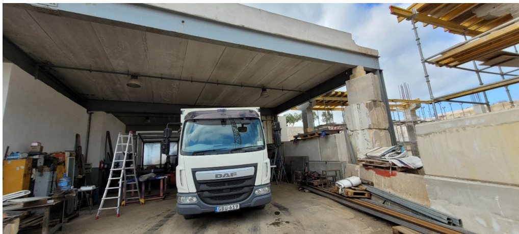
Figure 47 -- Street Level; Existing portal frame structure
