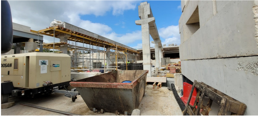
Figure 48 – Street Level – Second portion under construction
