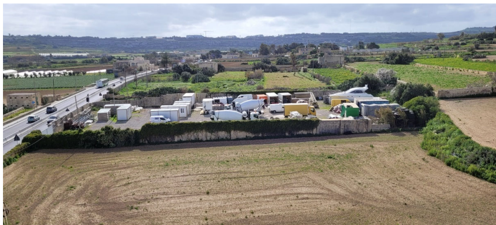
Figure 52 – Elevation of the Storage area of the Property as seen from Bonnici House
